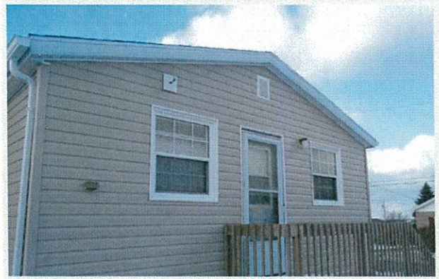
Figure 1- Before and after pictures of upgrades made to a home. Exterior repairs included new siding, eaves troughs and new screen door.
