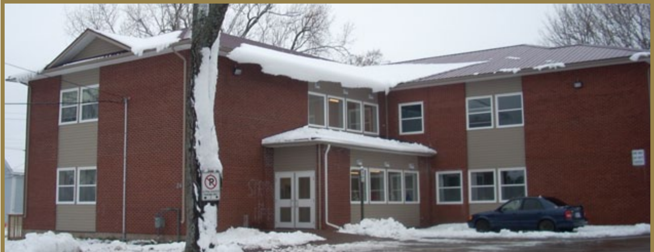
Amherst - A former office building was converted into 13 new affordable housing units.
