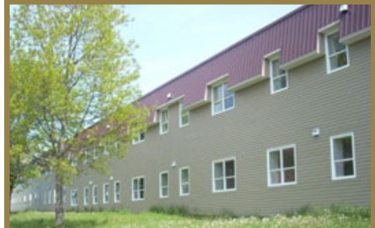
Amherst - These photographs show the dramatic conversion from a vacant school to 30 affordable rental housing units
